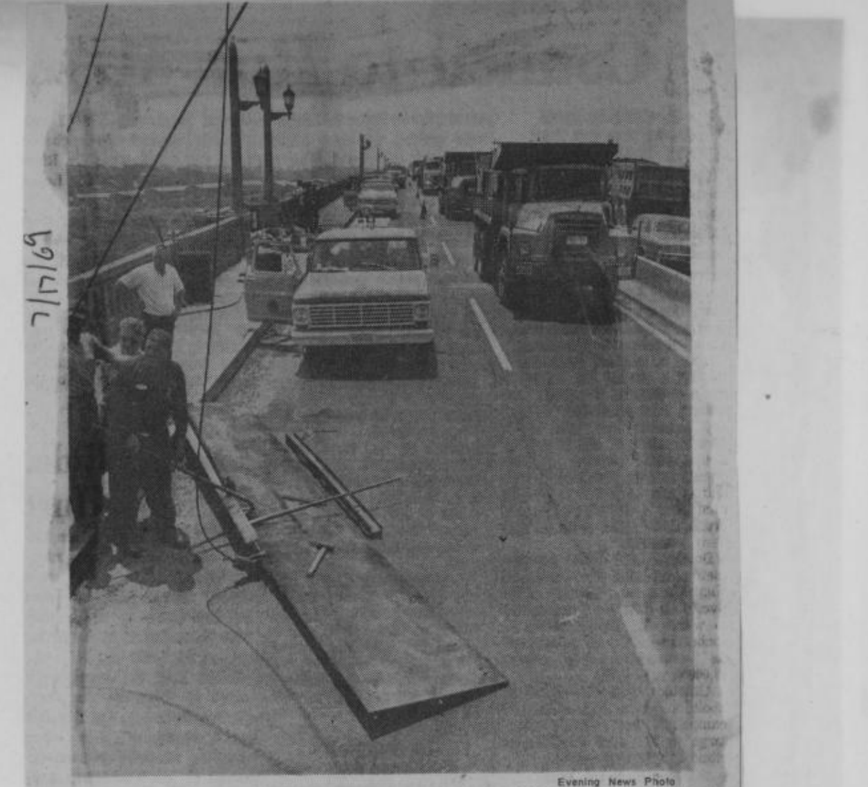
BRIDGING A PROBLEM — Traffic moves slowly in one north bound lane of Morris Goodkind Memorial Bridge as crews work on temporary repairs.
