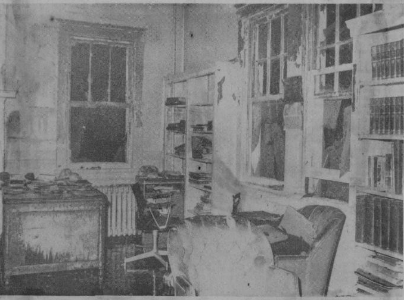
GUTTED—An office in Neighborhood House on Commercial Avenue was heavily damaged last night, when a fire of suspicious origin erupted at 10:55 p.m. Three hours
