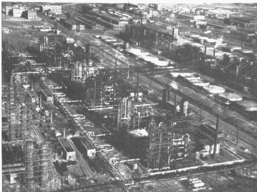
STANDARD OIL REFINERY, BAYWAY
