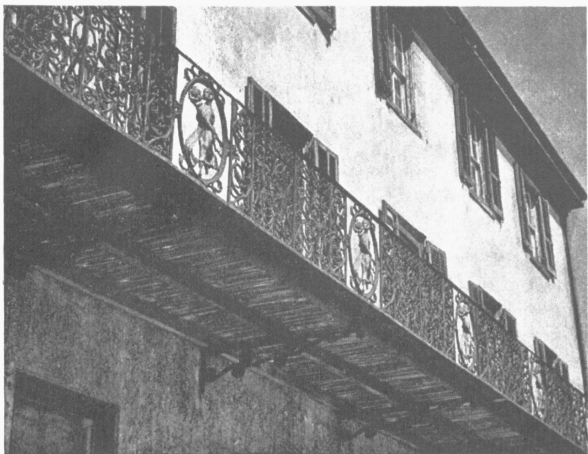
WROUGHT IRON BALCONY ON COLONIAL APARTMENTS, BORDENTOWN
