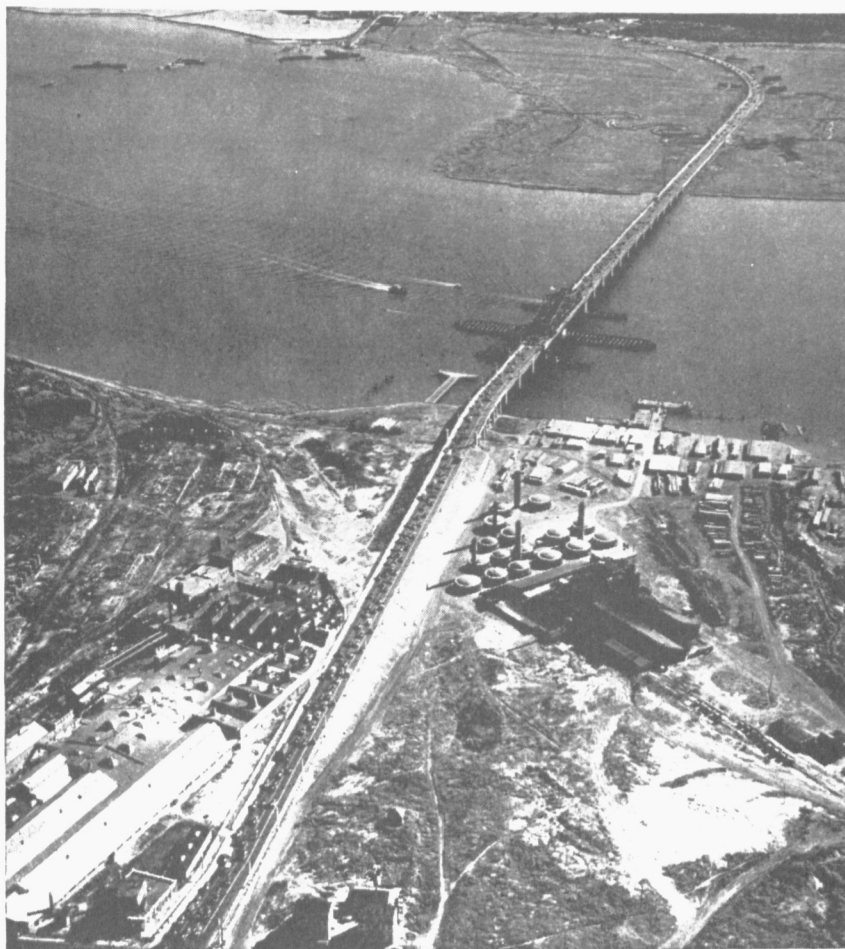
THE RARITAN RIVER AT PERTH AMBOY
