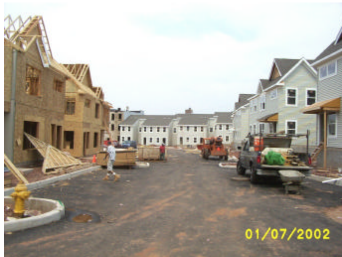
Hope Manor under construction
