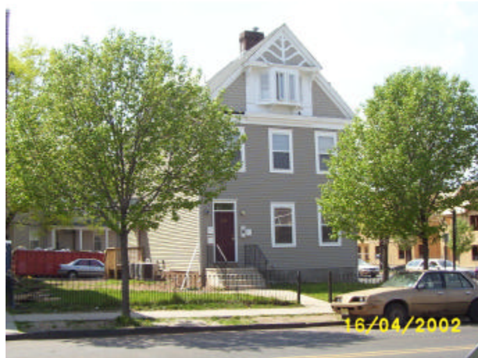
The first (multi-family) house to be rehabbed in Phase I
