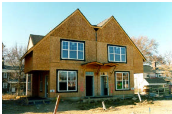
Wellington Ridge (under construction)
