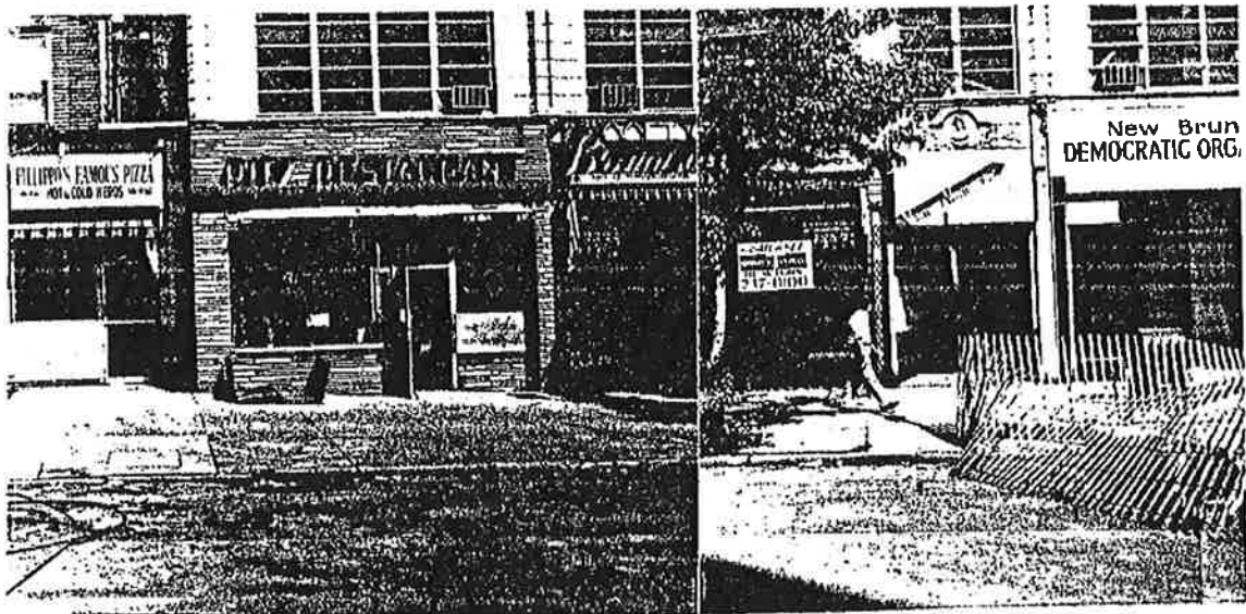
Livingston Avenue -- future mall extension
