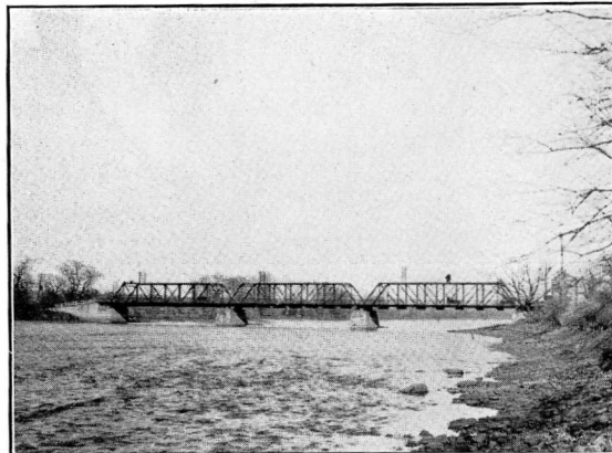
Landing Lane Bridge.
