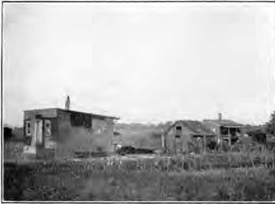
In a neighboring suburb—the results of no municipal control whatever, no supervision over subdivisions, no building code, no zoning.
