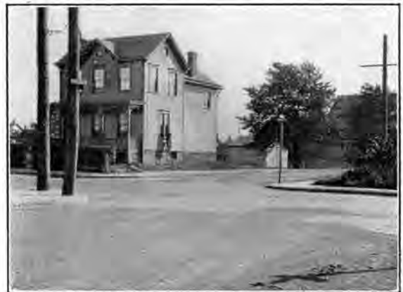
An offset street is a dangerous traffic trap.
