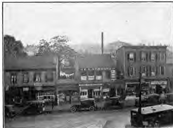
These buildings would be taken on Albany Street in extending Easton Avenue to Livingston Avenue.
