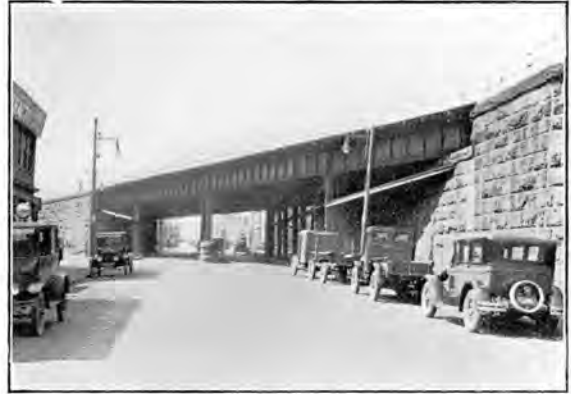
French Street looking west under the Pennsylvania tracks.
