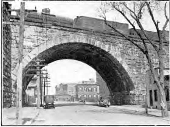
The Pennsylvania Railroad arch over Neilson Street.
