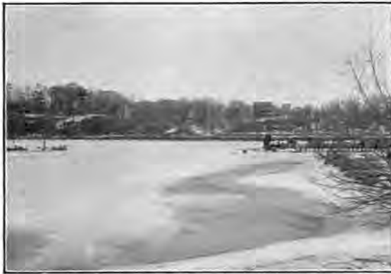
Looking across the Raritan River towards the Highland Park terminus of the proposed bridge. Note the high bank of the river as well as the undeveloped condition of the ground.
