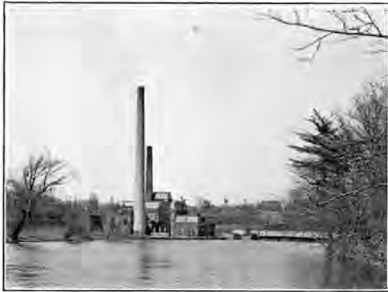
New Brunswick pumping station.
