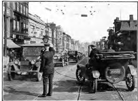
Obstruction caused by left hand turns at Albany and George Streets.
