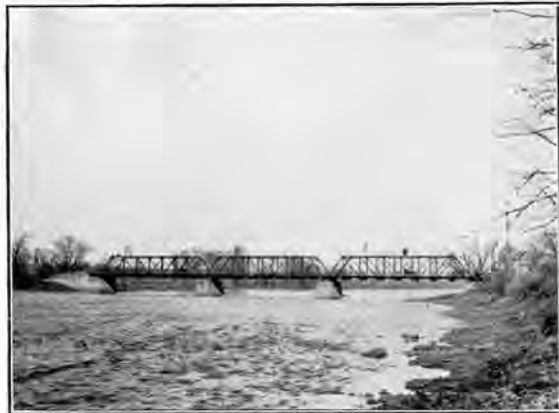
Landing Lane Bridge.
